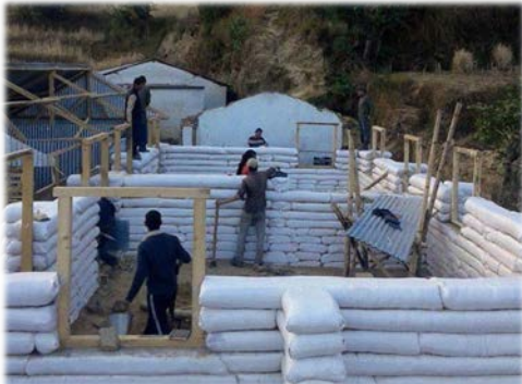
Earthbag Construction, Makwanpur, Nepal
