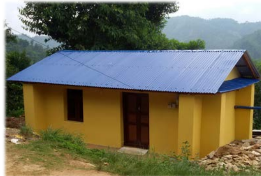
Completed Earthbag House, Gorkha, Built by Good Earth Nepal
